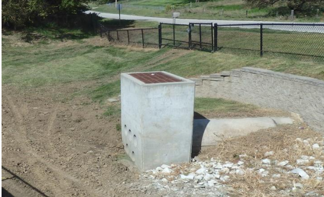
North Pond Discharge Structure
