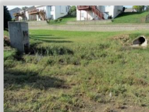
Figure 5.1 – Wet basin grass & weeds at Tipton inlet
