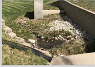
Figure 6.3 – North Pond Outlet
