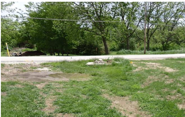
Figure 5 – May 2019; Easement Spillway Discharge
